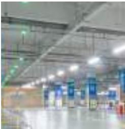
Indoor structures, underground parking area
