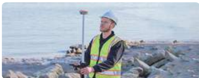
Building Foundation Stakeout
