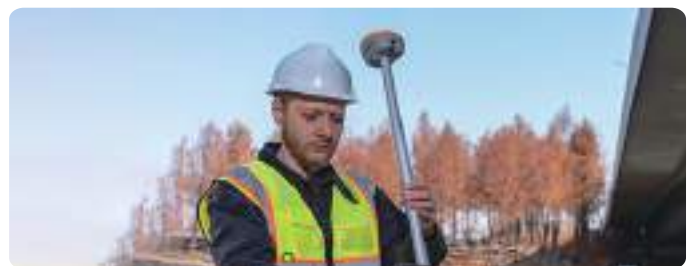
Construction Site Stakeout
